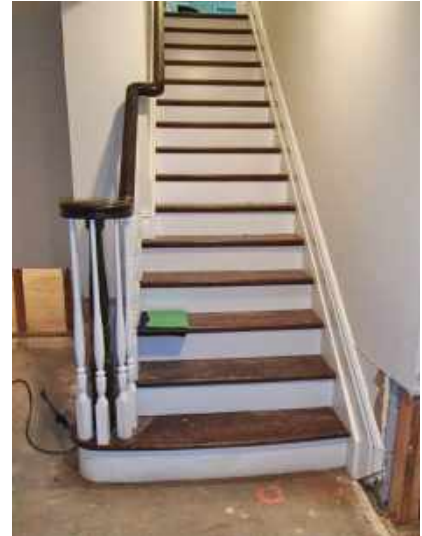
▲ Finished stairs are not covered.
