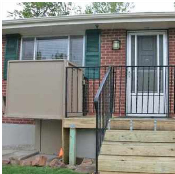
▲ An insured chair lift attached directly to a building or covered 4x4 16 SF landing.
