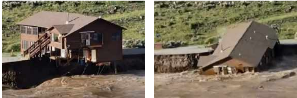
▲ A structure experiences sudden erosion during Yellowstone flooding in 2022.
