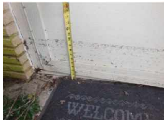
▲ Example of a good photograph: clear picture of the waterline with measurement.
