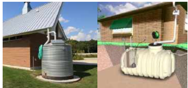
▲ Non-insured cisterns outside (l) and underground (r)
